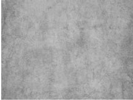
Pared de Cemento
